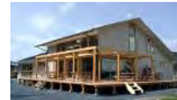
Eco Club House 1kW Fuel Cell 2 units
