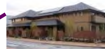
Hydrogen Fuel Cell Demonstration Home 1kW Fuel Cell 7 units
