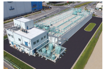
Minami-Honmoku Block #5 wastewater treatment facility
