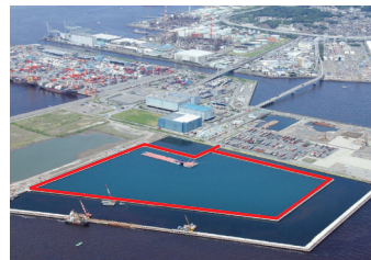
Minami-Honmoku Block #5 Final Disposal Site
