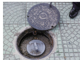
Manhole for direct sewage portable toilet
