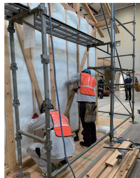
断熱施工の実技講習
