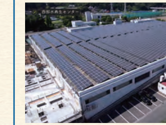
▲ Electricity generated from the tops of facilities is sold to power companies.
