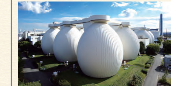
▲ Digestion tank at a sludge treatment plant
